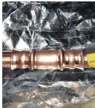
After the pressing cycle is complete, the double circular bands can be seen on each end of the RLS fitting.
