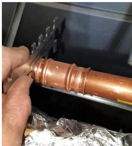
*The RLS crimp gauge fits over the crimp band to quickly confirm that a reliable joint has been made.*
