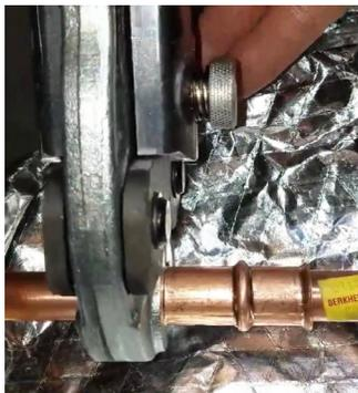
The RLS press tool can fit into tight spaces where brazing would be difficult and/or dangerous.
